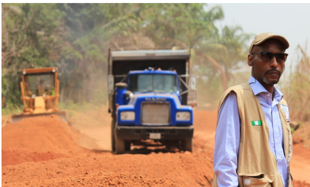
Construction Supervision at Enugu, World Bank RAAMP
