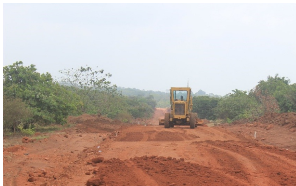
Construction Supervision at Enugu, World Bank RAAMP
